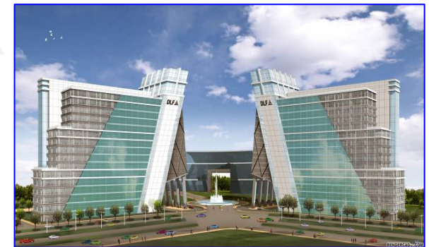
Building No 9, Cybercity, Gurgaon – Block B 0.76 msf
