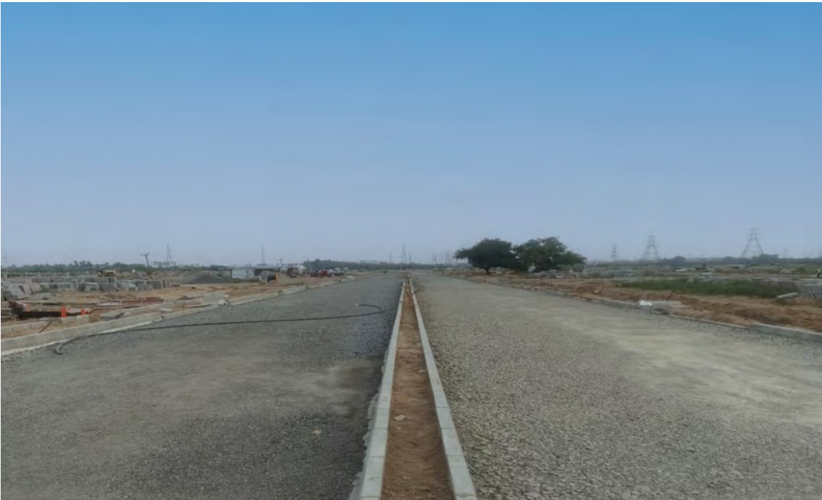
Parc Estate internal roads under development in Chennai
