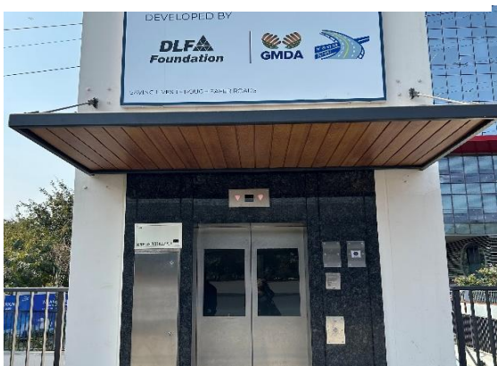
Lift installed at Subway-B
