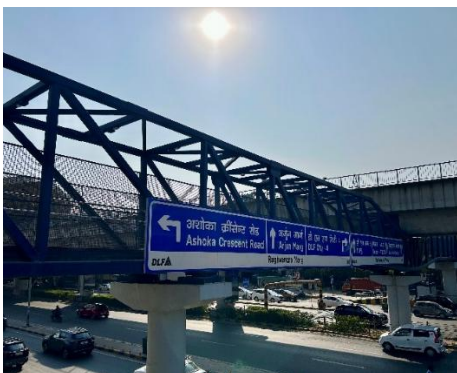
View of Foot over bridge on approach to Ashoka
