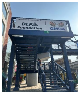
Foot over bridge-1
