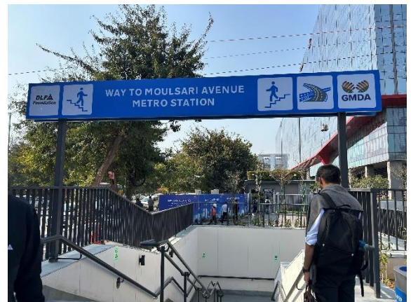
Entry to the Pedestrian Subway
