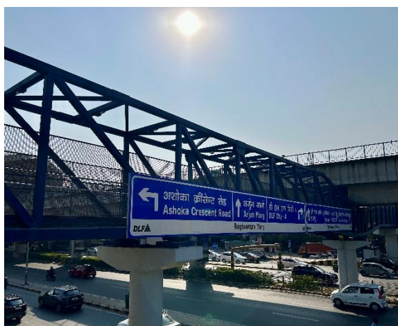
View of Foot over bridge on approach to Ashoka Crescent
