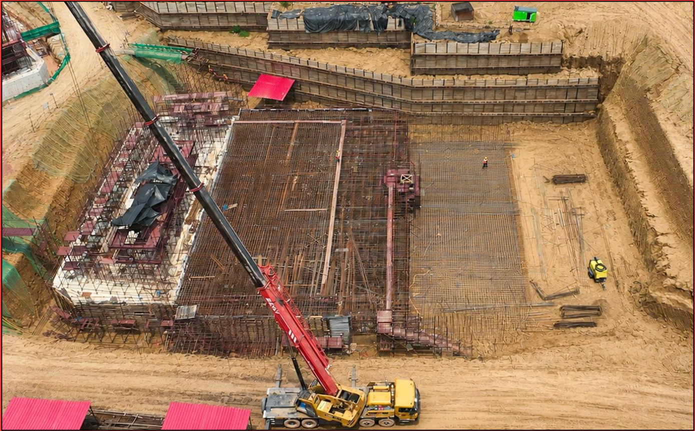
Tower E Raft Reinf. Work in Progress
