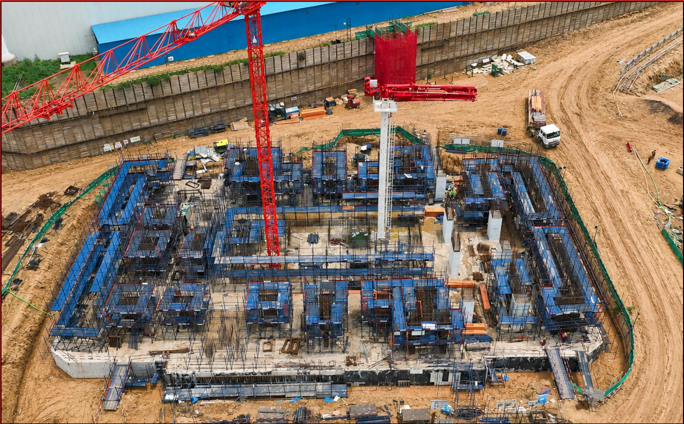
Tower C B3 Level Work in Progress
