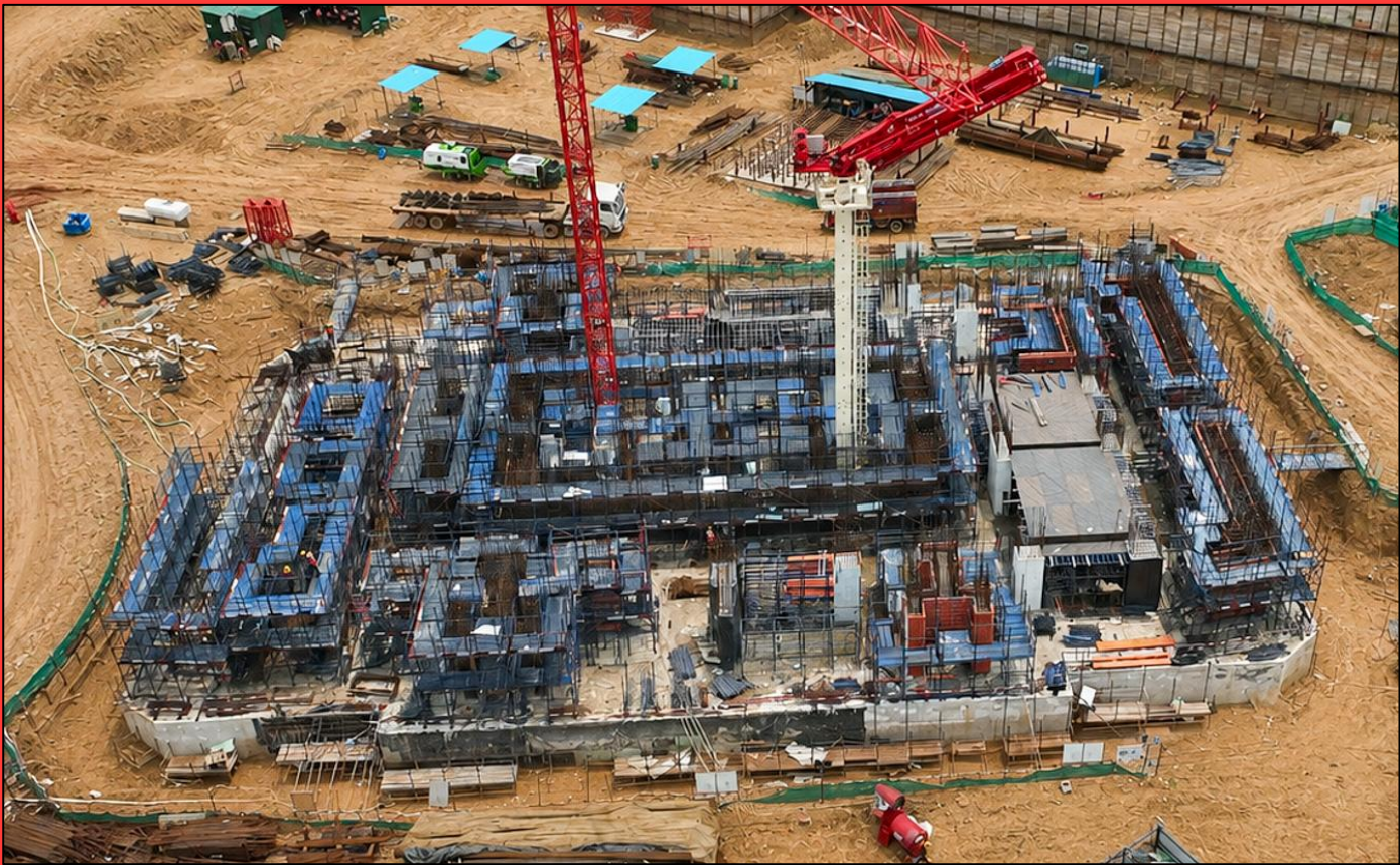
Tower B B3 Level Work in Progress
