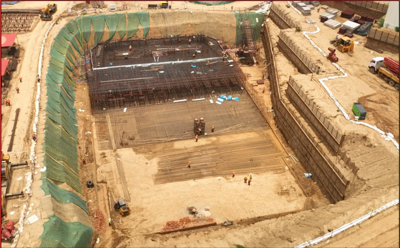
Tower E Raft Reinf. Work in Progress
