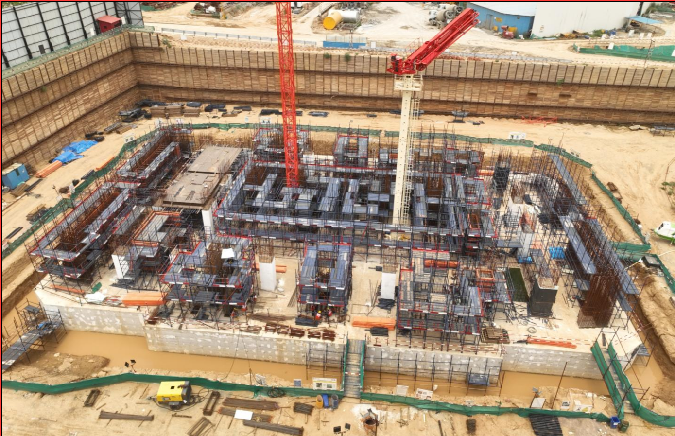
Tower A B3 Level Work in Progress
