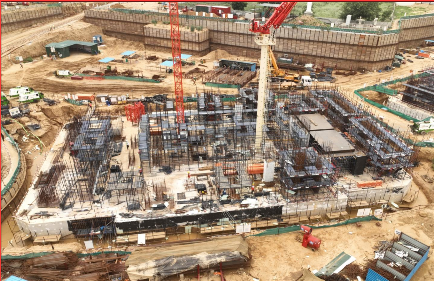
Tower B B3 Level Work in Progress
