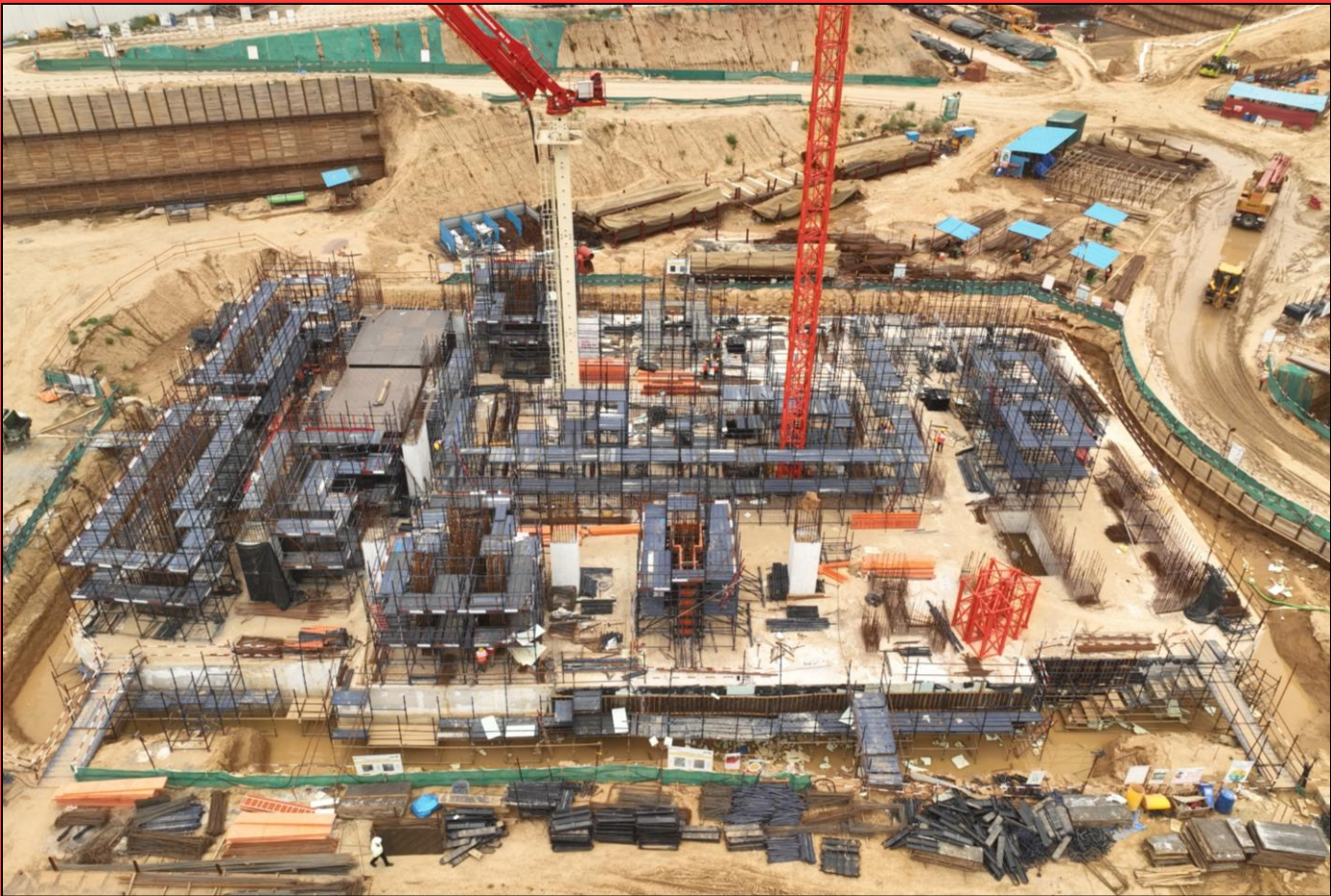
Tower C B3 Level Work in Progress
