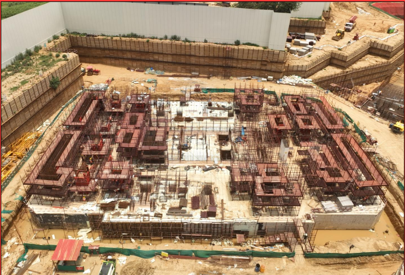
Tower F B3 Level Work in Progress
