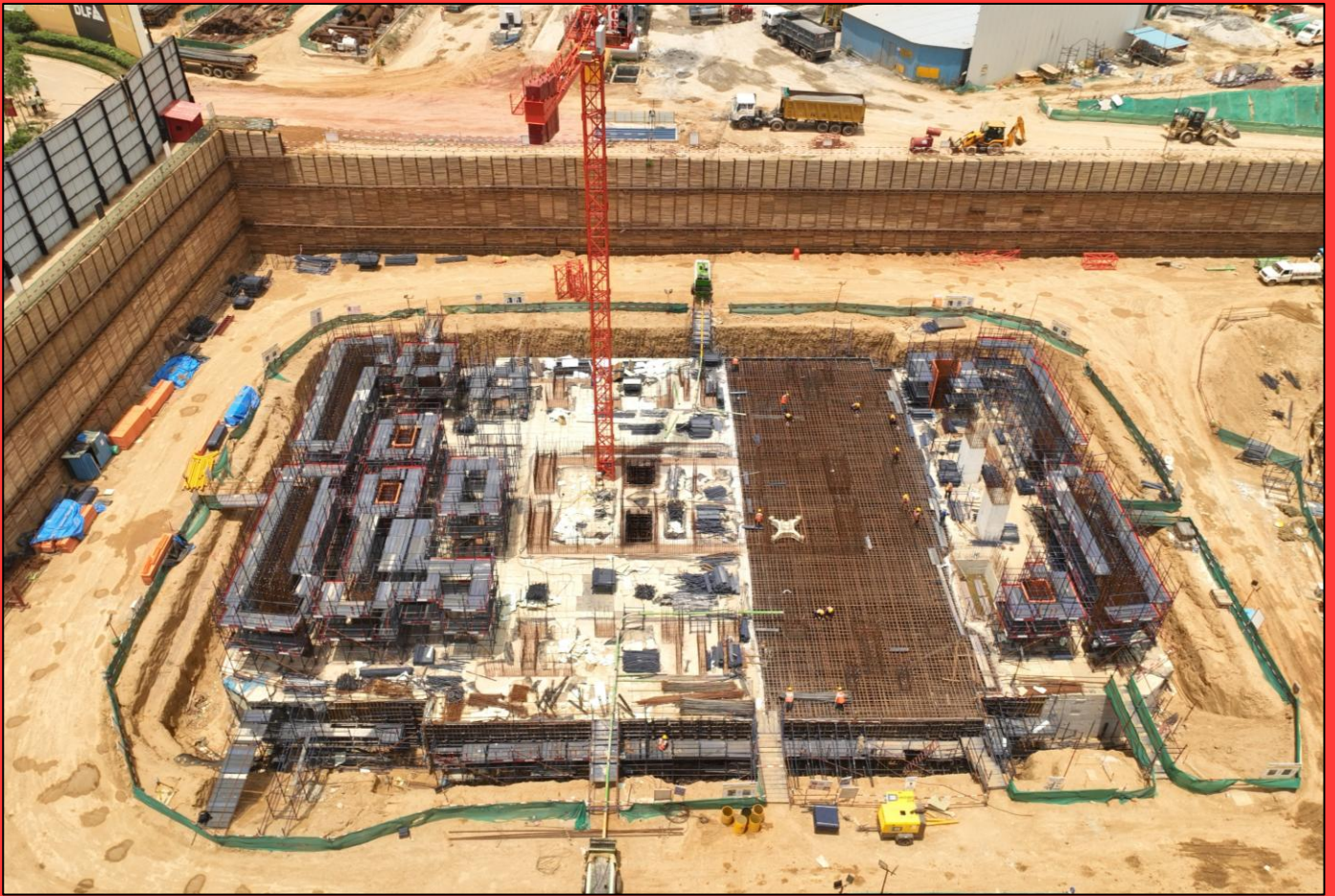
Tower A Raft & Vertical Reinforcement Work in Progress
