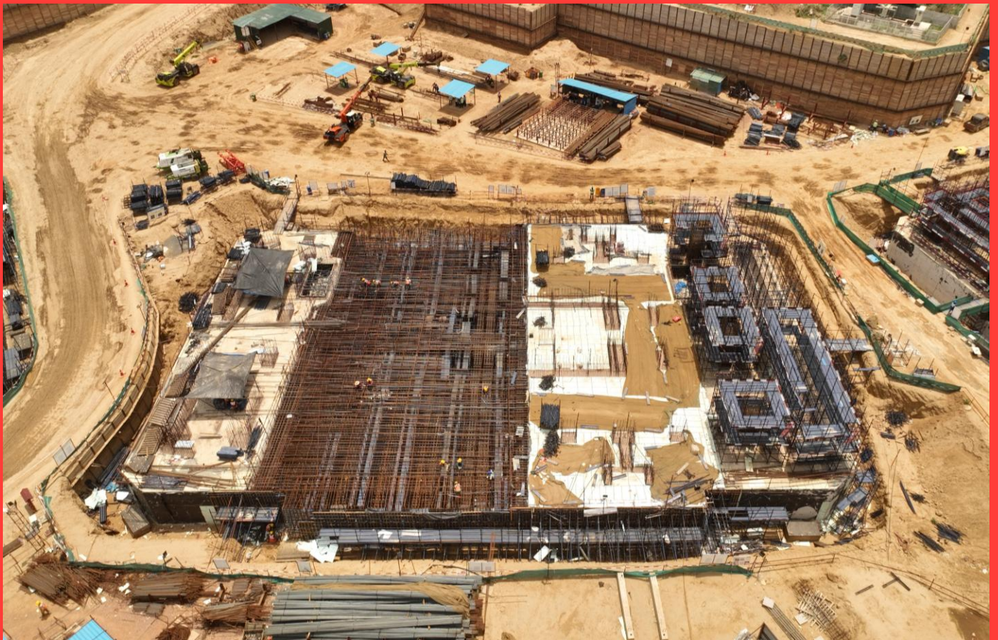
Tower B Raft & Vertical Reinforcement Work in Progress
