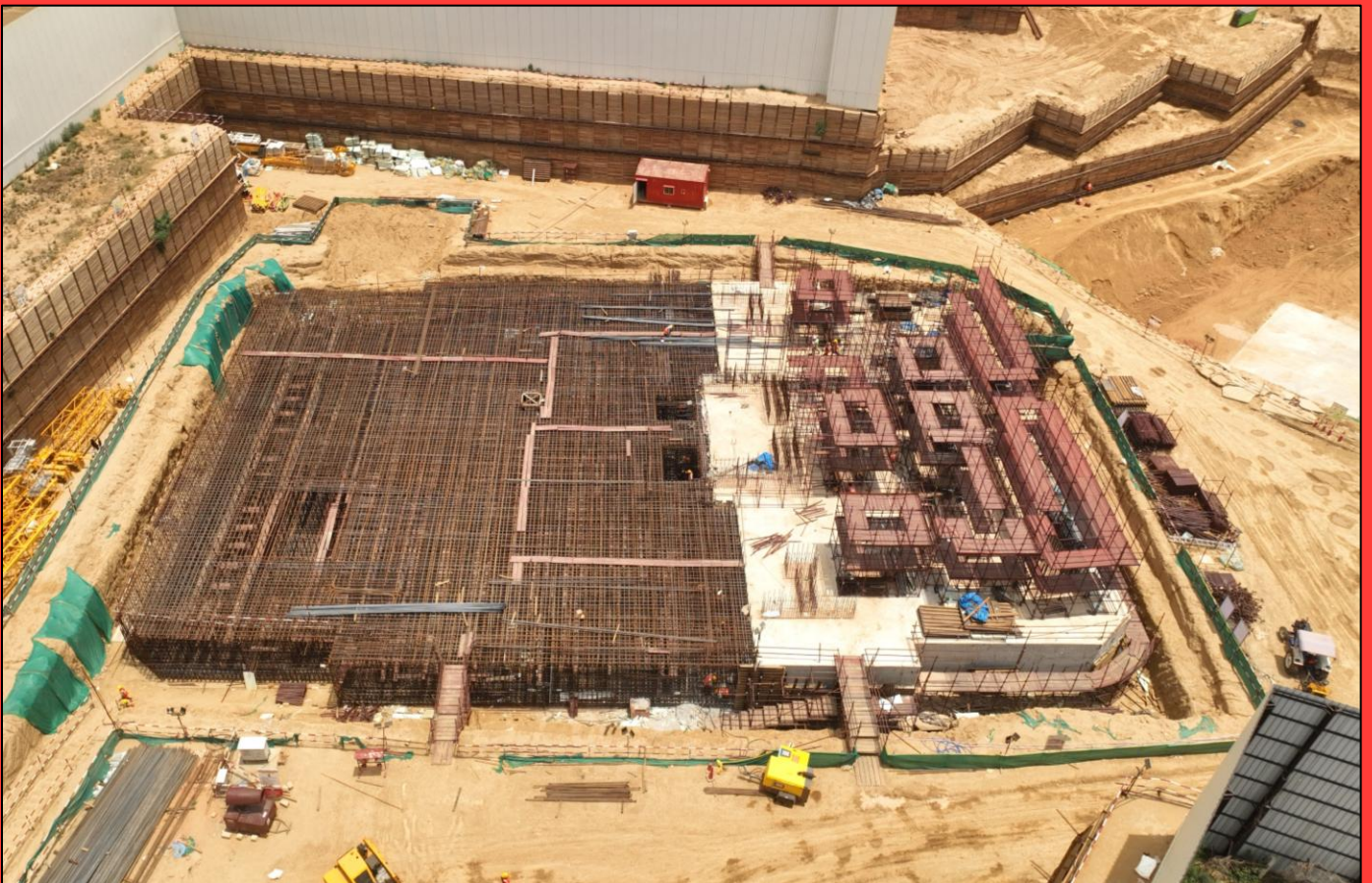
Tower F Raft Reinforcement Work in Progress
