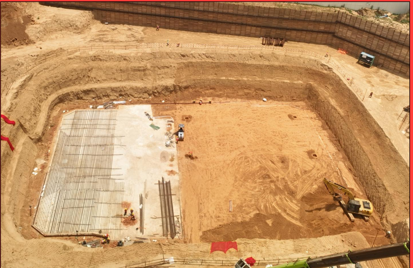
Tower D Foundation works commenced
