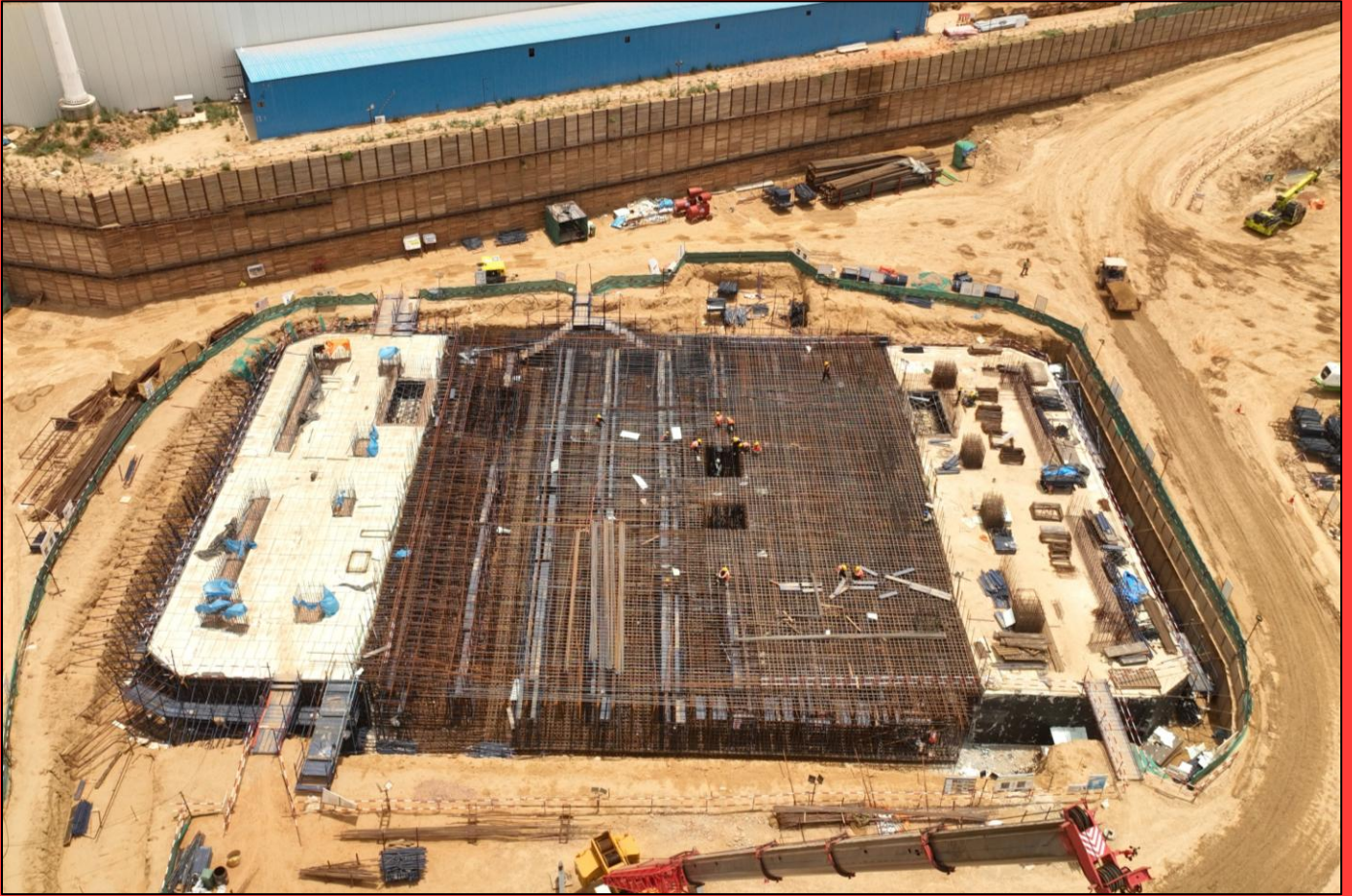
Tower C Raft & Vertical Reinforcement Work in Progress
