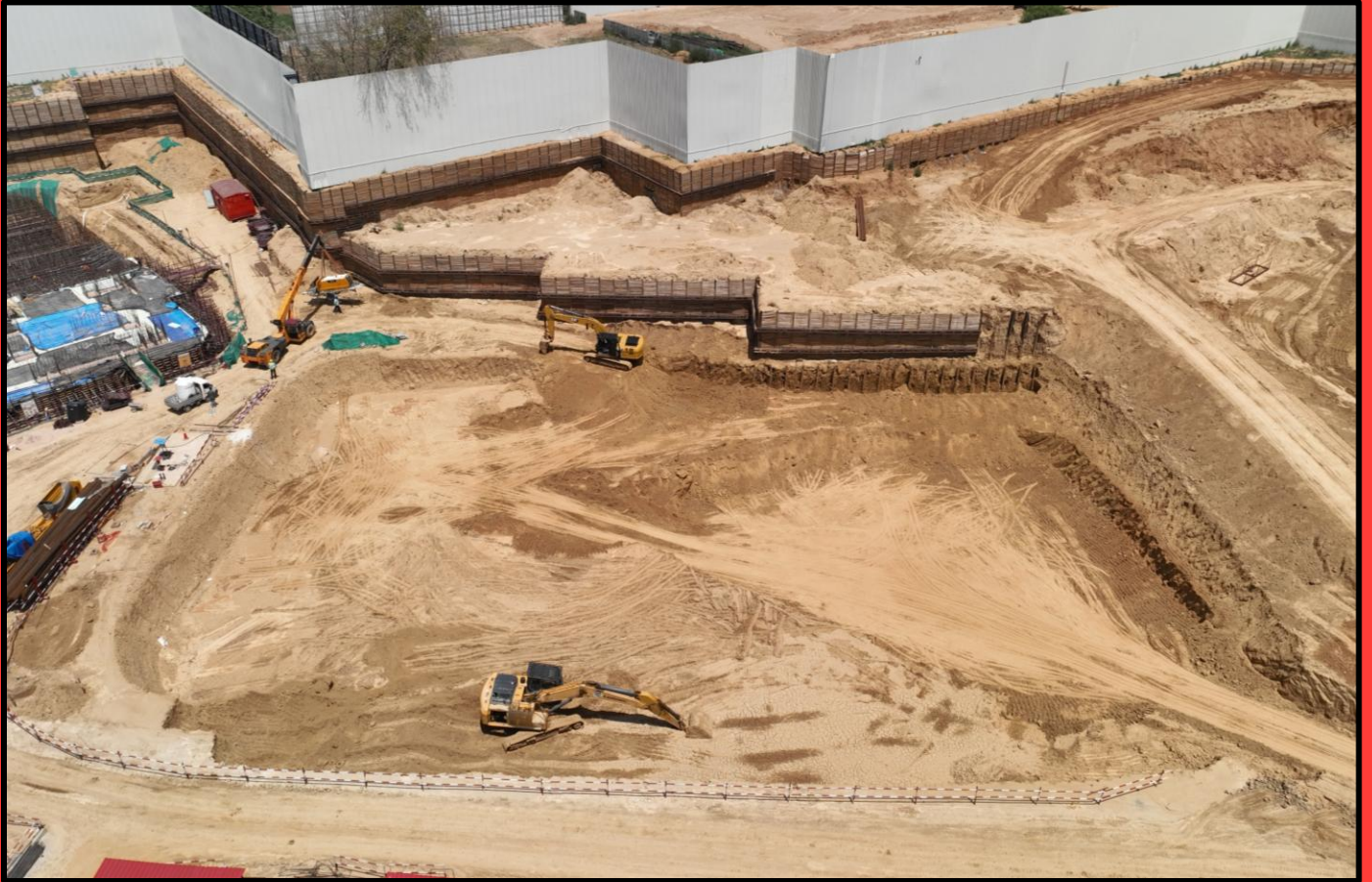
Tower E Shoring Work in Progress
