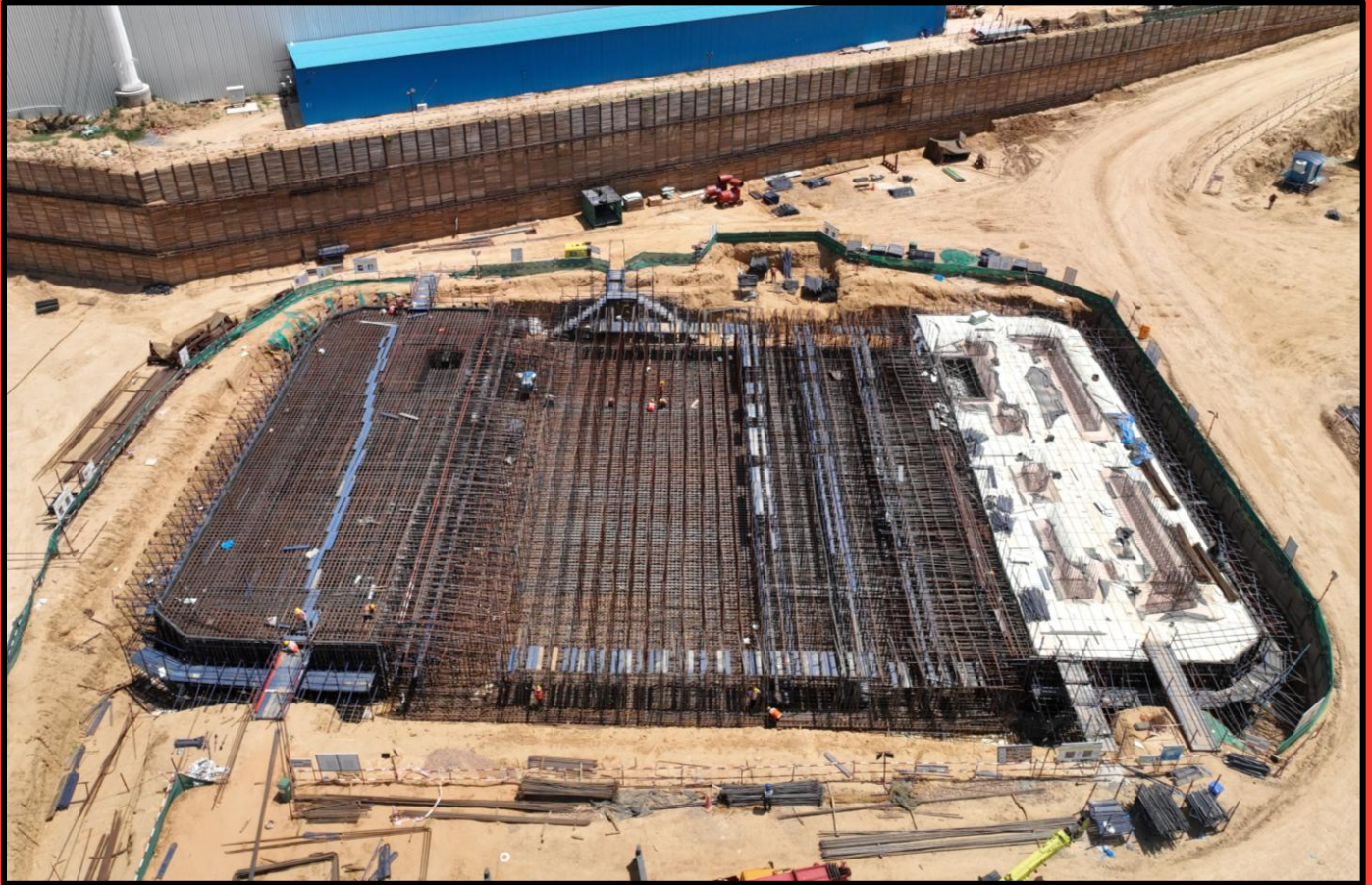
Tower C Raft Reinforcement Work in Progress
