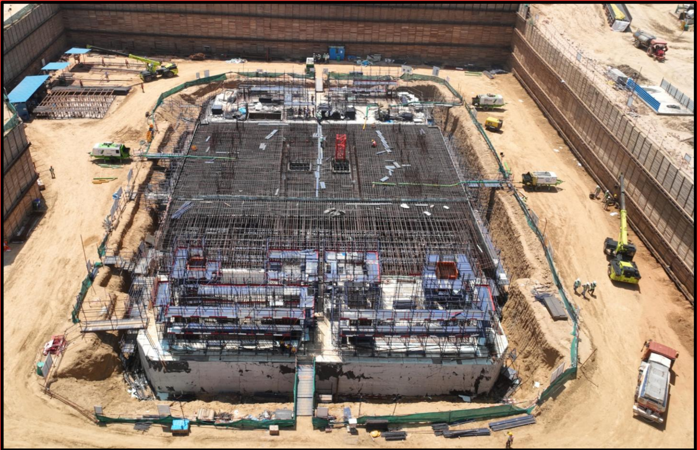
Tower A Raft & Vertical Reinforcement Work in Progress
