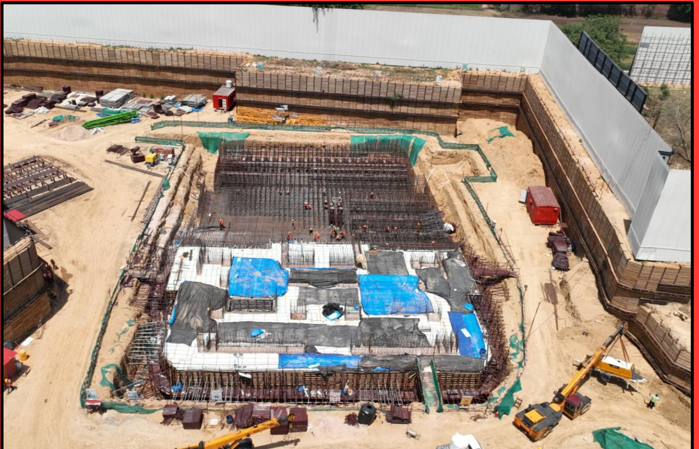
Tower F Raft Reinforcement Work in Progress
