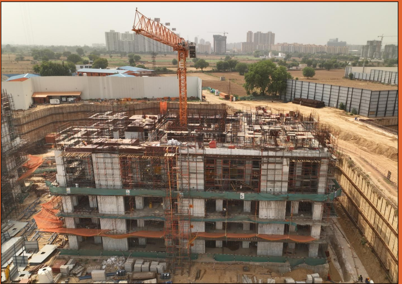
Tower E 1 st Floor column casting Work in progress
