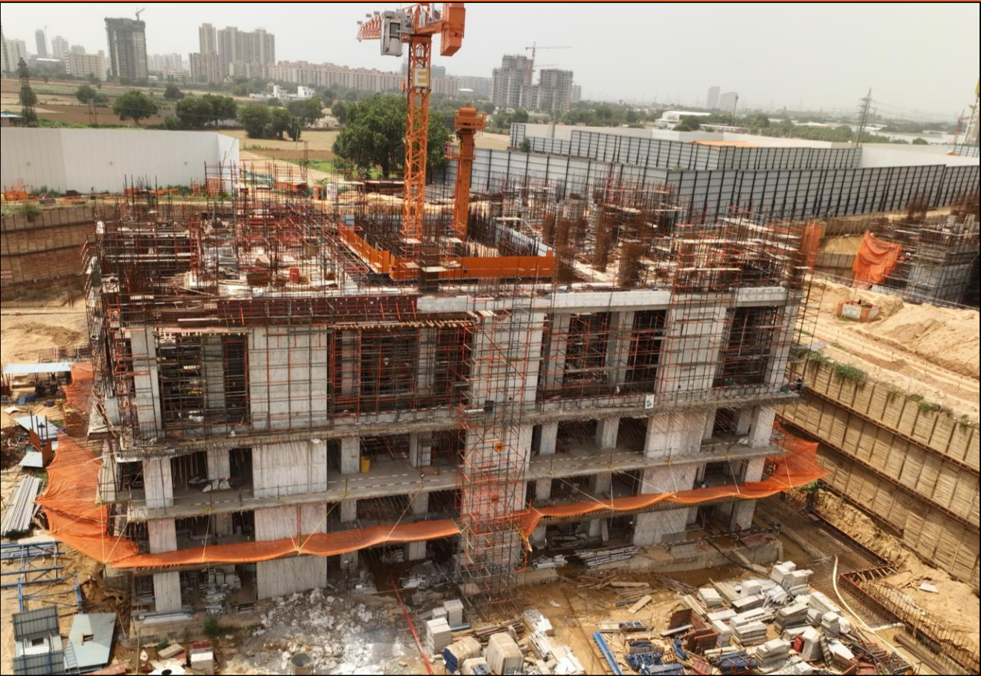
Tower E 1 st floor slab completed
