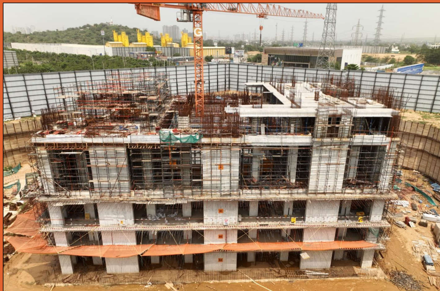
Tower G 1 st Floor Slab casting Work in progress
