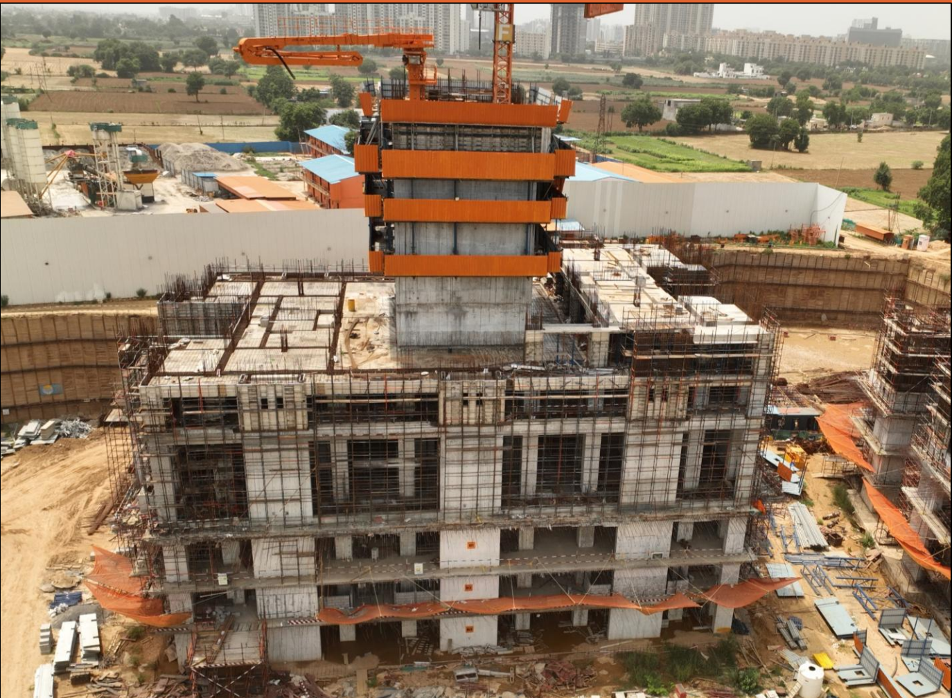
Tower F 6 th Floor Core wall Casted, 1 st Floor Slab Completed
