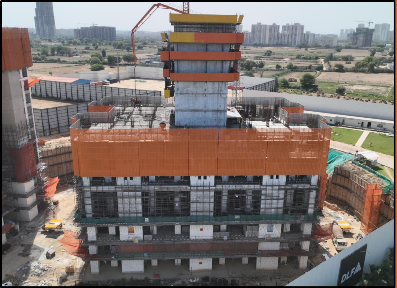
Tower A 9 th Floor core wall casted, 3 rd Floor slab completed.
