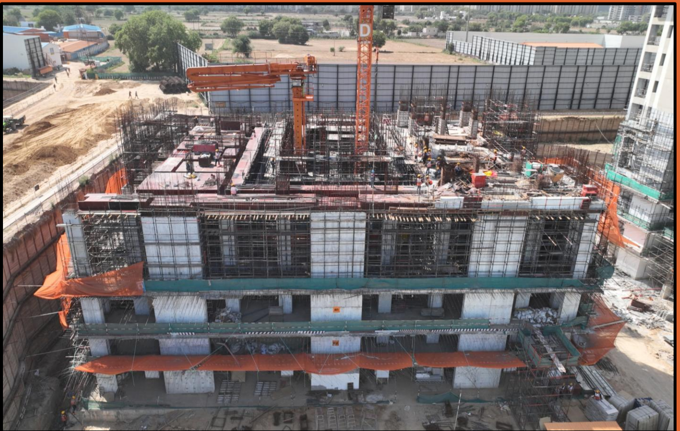
Tower D 1 st Floor column casting WIP
