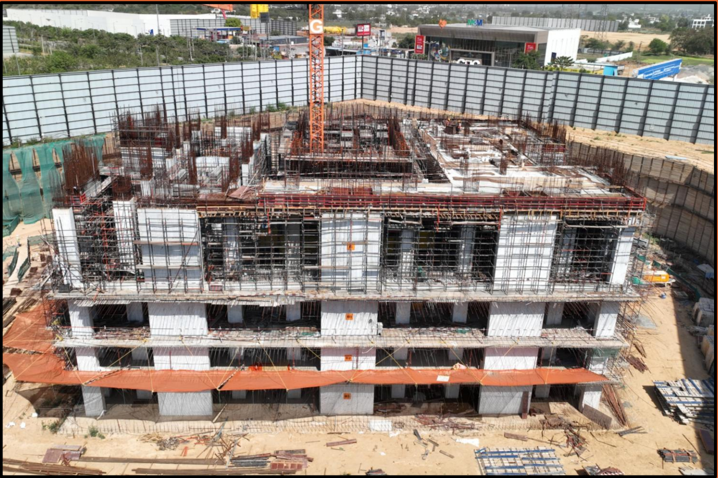
Tower G 1 st Floor column casting Work in progress
