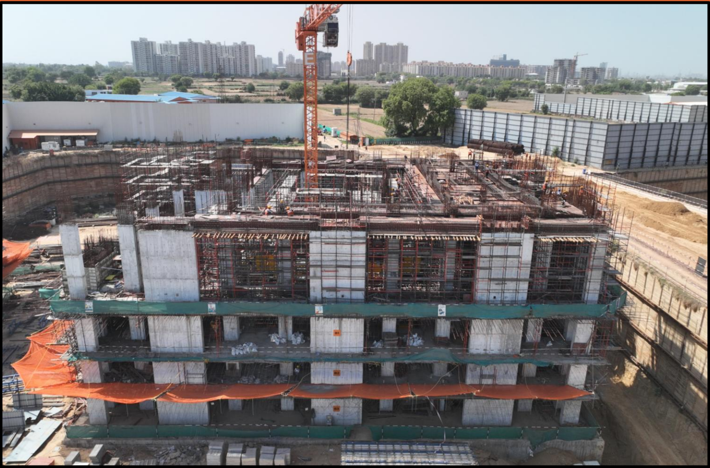
Tower E 1 st Floor column casting Work in progress
