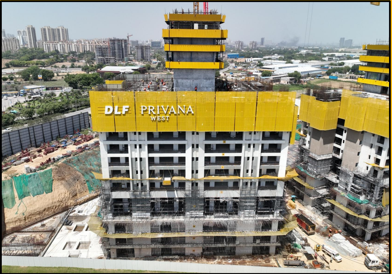
Tower A 12 th Floor core wall casted, 8 th Floor slab completed
