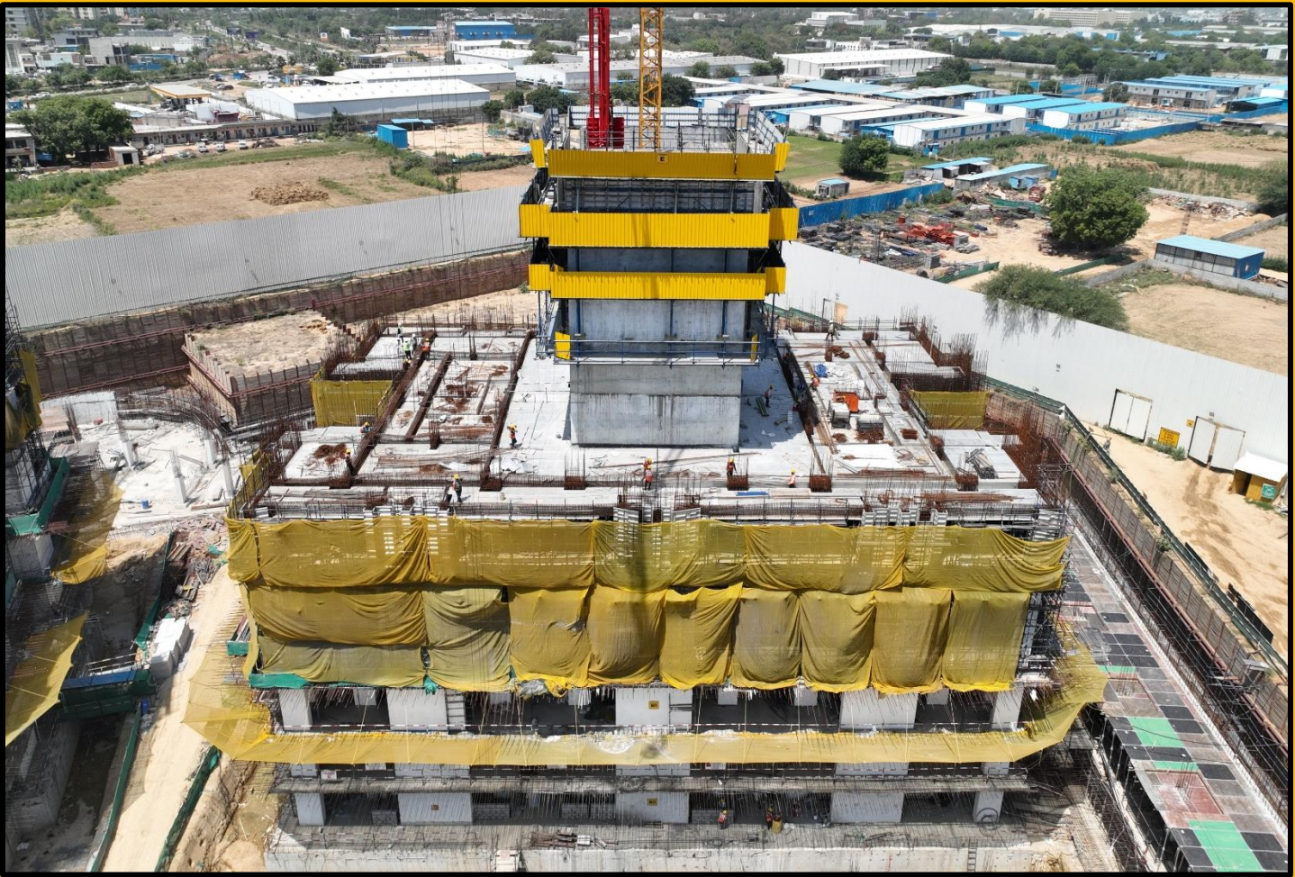
Tower E 6th Floor core wall casted, First Floor slab completed
