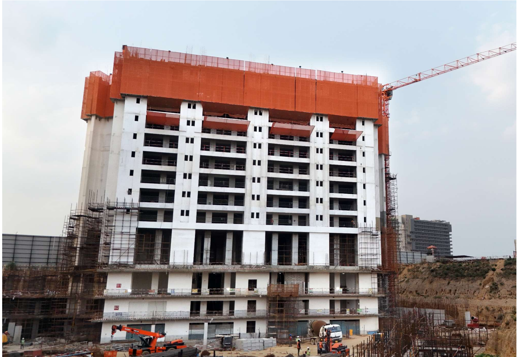
Tower C – 10F Slab WIP
