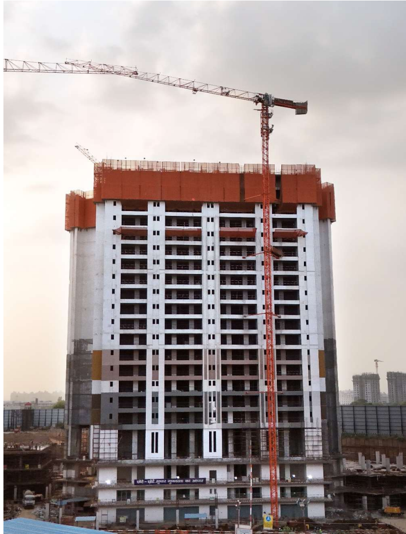
Tower B – 19F Slab WIP
