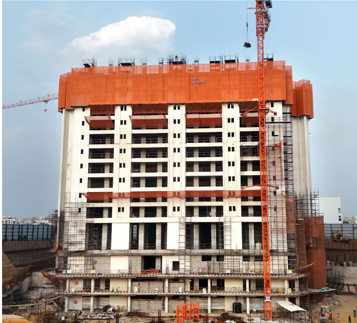
Tower D – 12F Slab WIP
