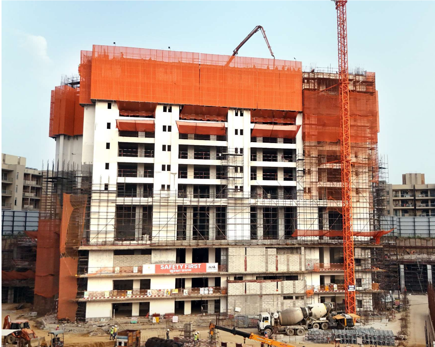
Tower E – 8F Slab WIP
