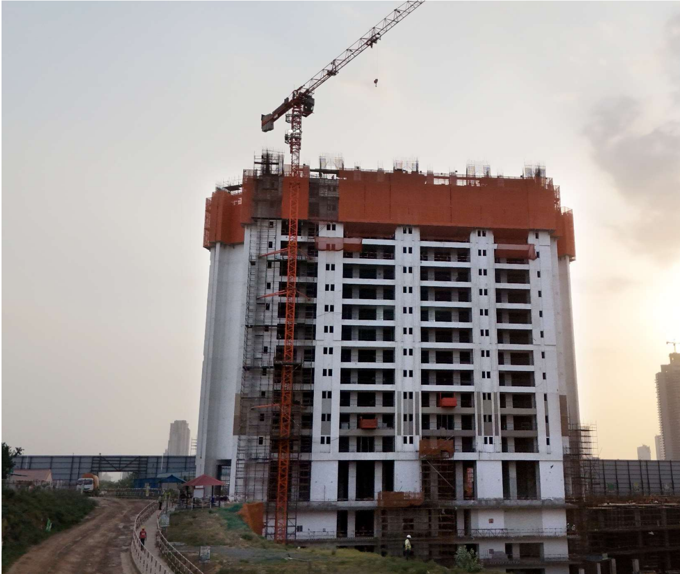
Tower A – 16F Slab WIP
