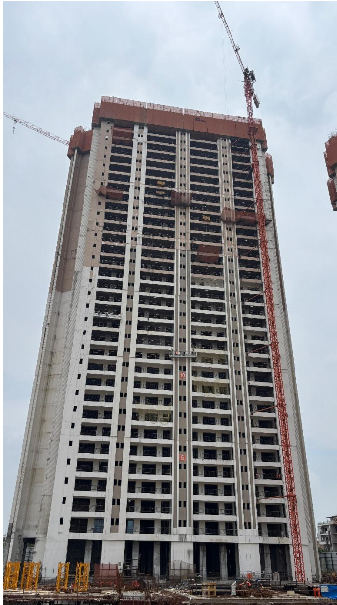
Tower D – 36F Slab WIP
