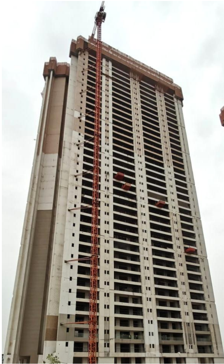
Tower A – Terrace Slab done
