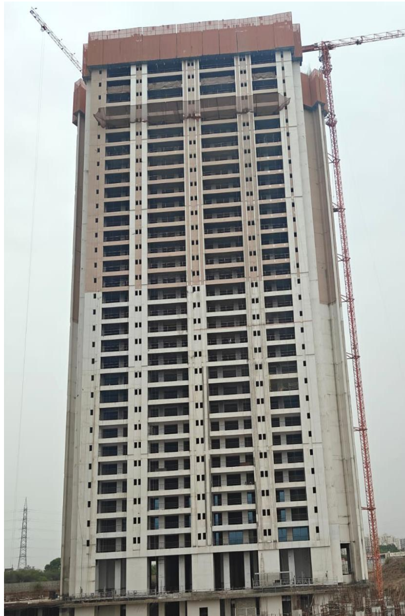
Tower C – 35F Slab WIP
