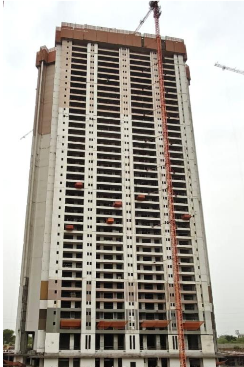
Tower B – Terrace Slab done
