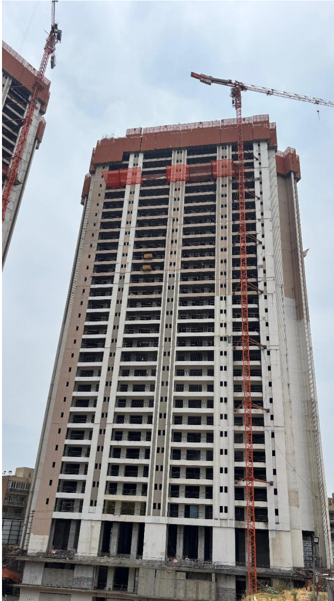
Tower E – 32F Slab WIP
