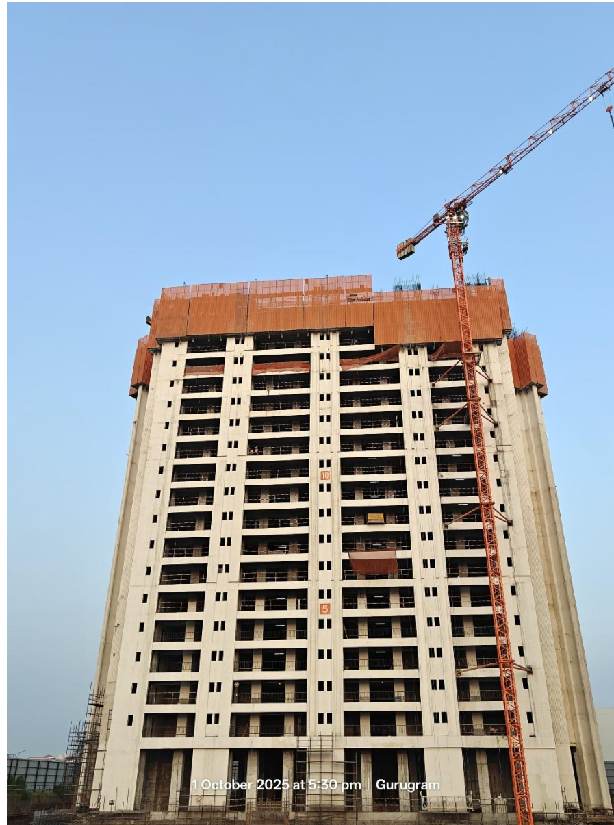
Tower D – 20F Slab WIP
