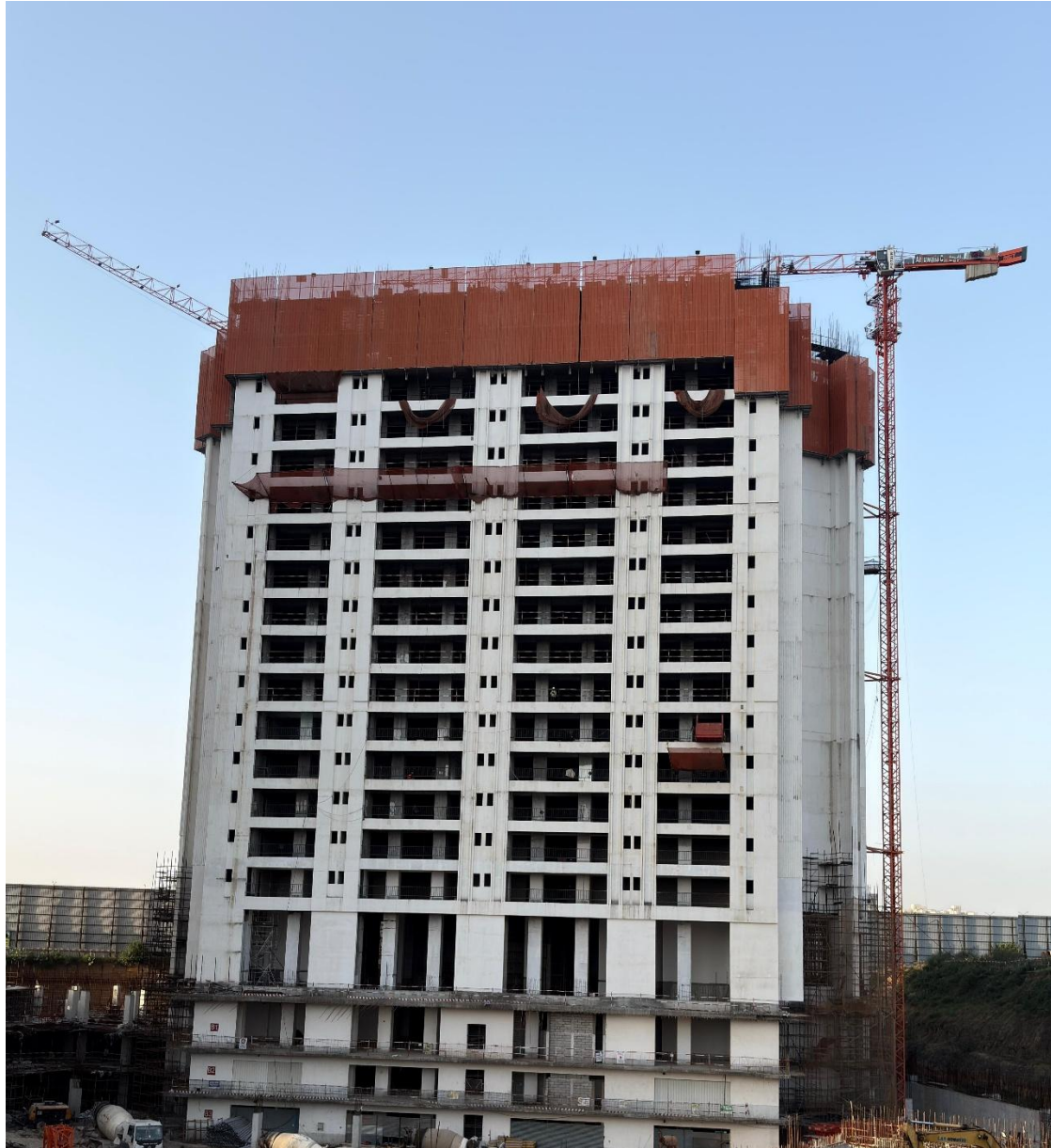
Tower C – 18F Slab WIP
