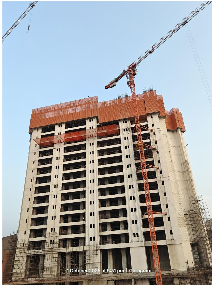
Tower E – 16F Slab WIP
