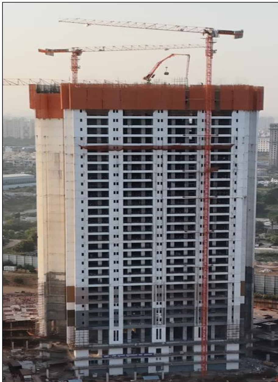
Tower B – 30F Slab WIP
