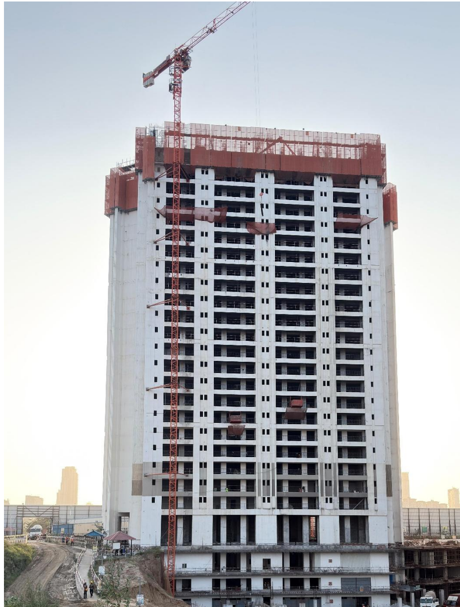
Tower A – 25F Slab WIP
