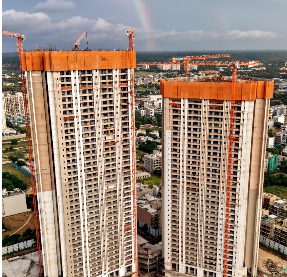
Tower D – Terrace Slab done, Tower E – 36F WIP
