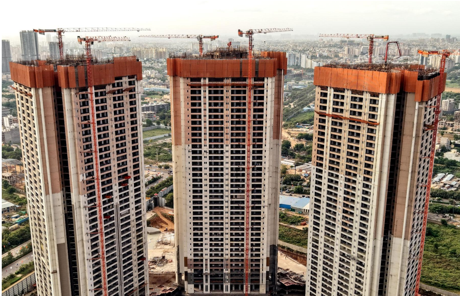
Tower A, B & C – Terrace Slab done
