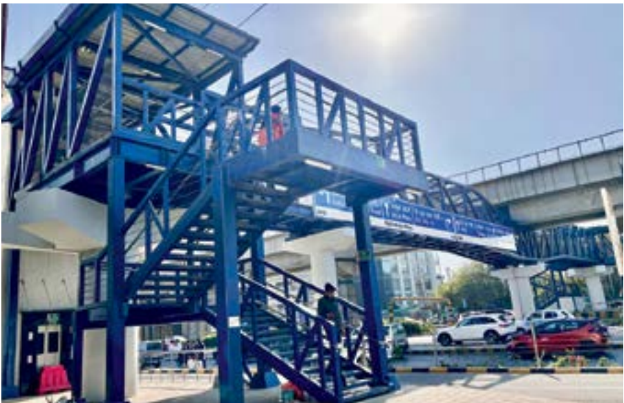
The newly constructed Public Foot-Over Bridge connecting Chakarpur village with SikanderpurAshoka Crescent Marg at Raghvendra Marg, Gurugram
